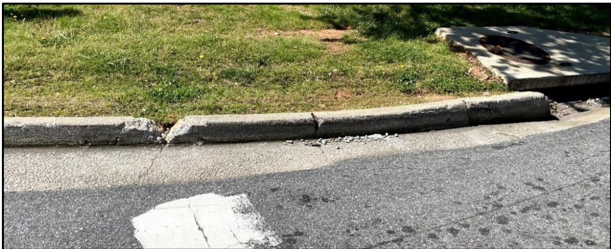
Figure 18: Curb and Storm Drain Damage at the Southwest Corner of the Intersection
