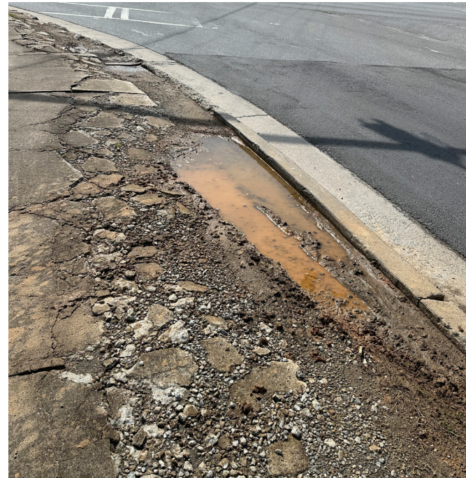
Curb Damage Present at the Intersection of McCollum Parkway and Big Shanty Drive
