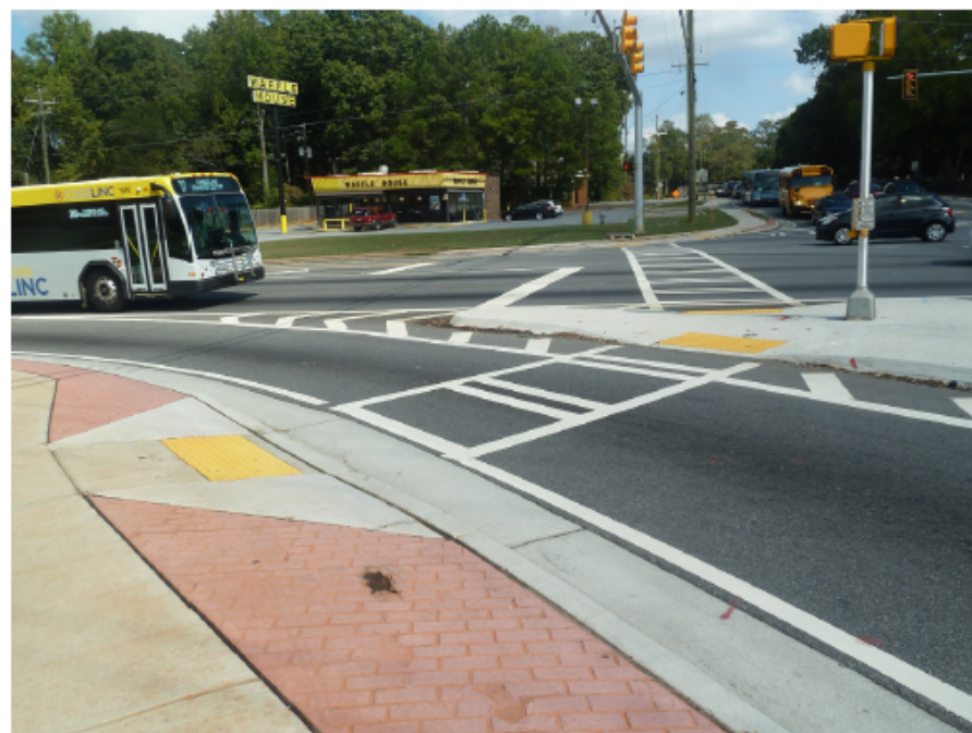
A long but accessible, marked, and signalized intersection.
