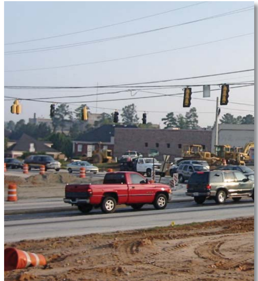
Road construction in Henry County.
