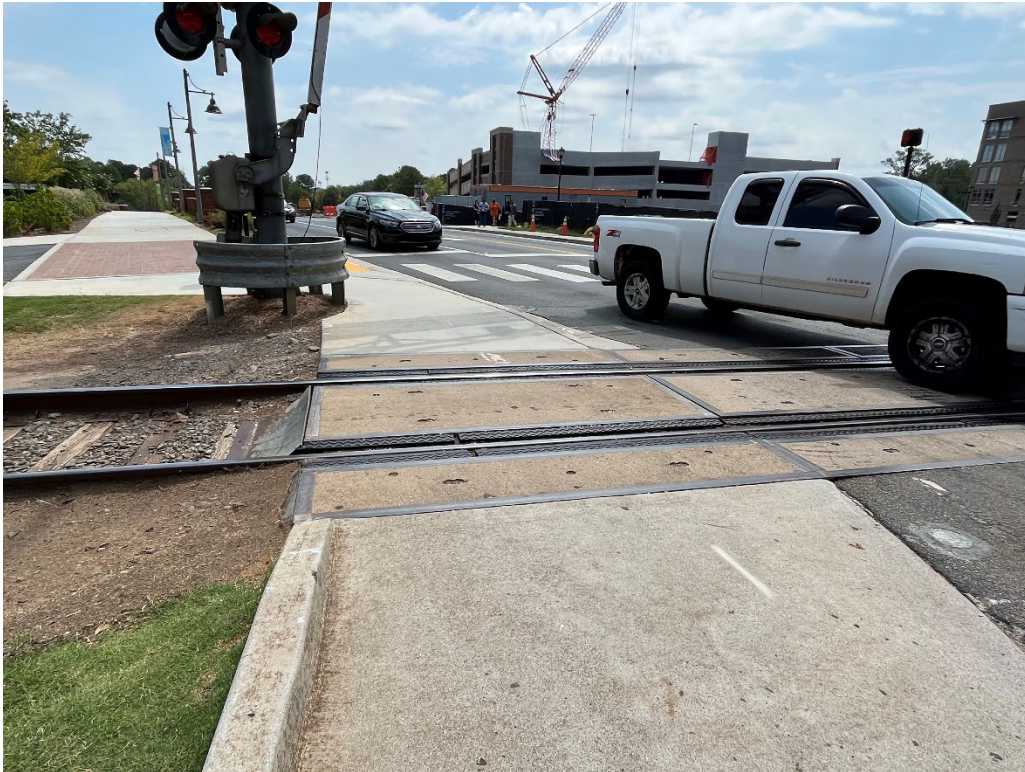
Figure 102: Pedestrian Railroad Crossing on Sidewalk in Woodstock, GA
