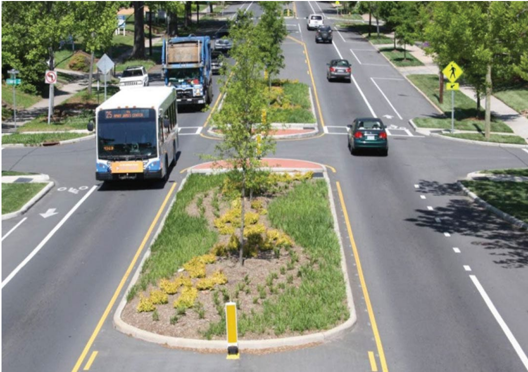
Figure 86: Arterial with Median and Pedestrian Refuge
