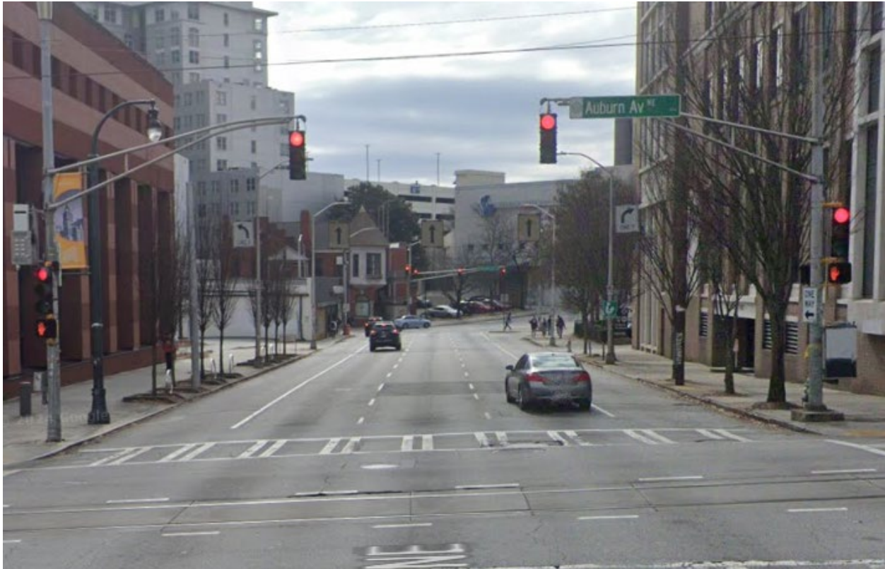
Figure 88: Supplemental Signal Heads on Pedestals in Downtown Atlanta
