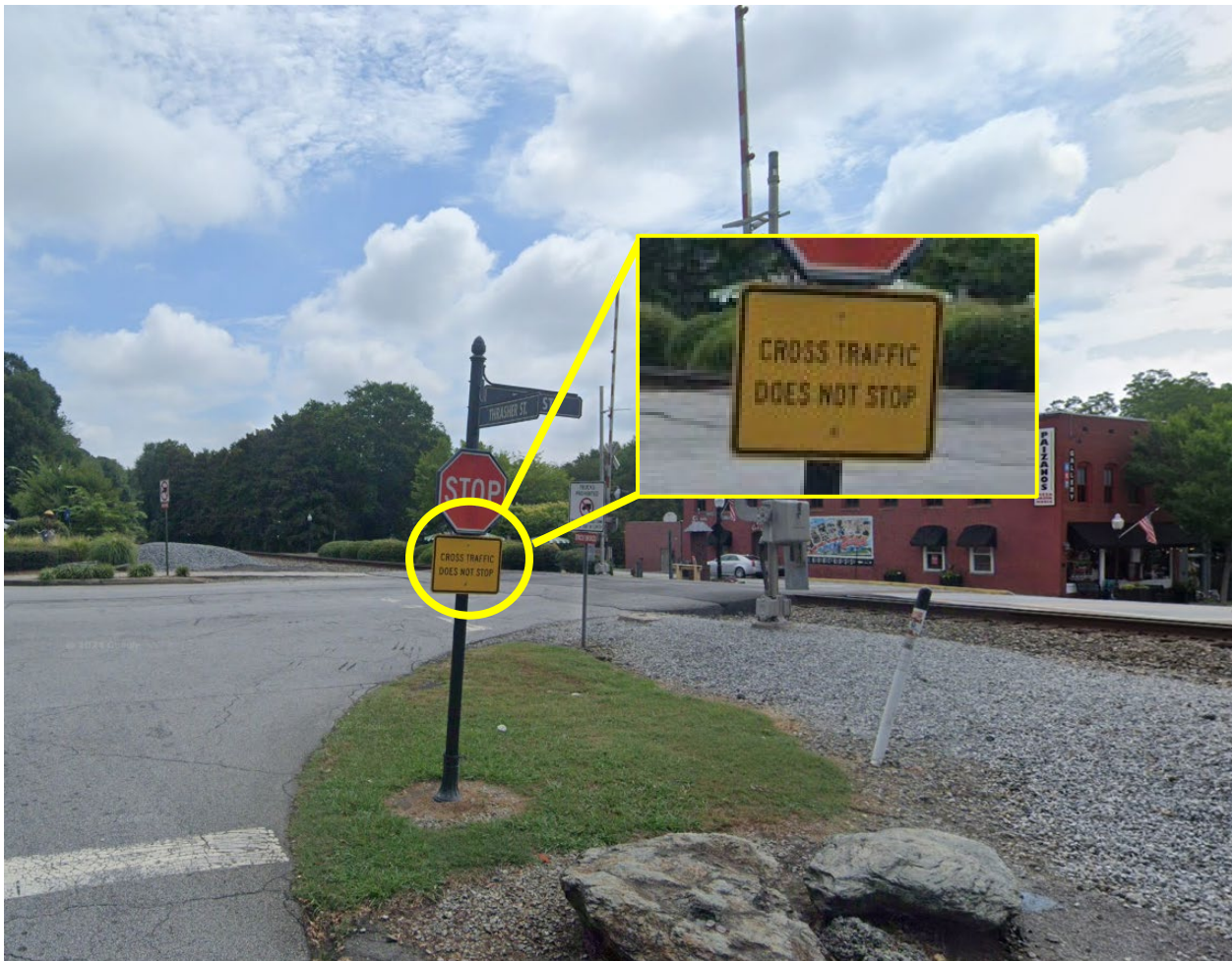
Figure 101: Proper Signage at Stop-Controlled Intersection near At-Grade Crossing
