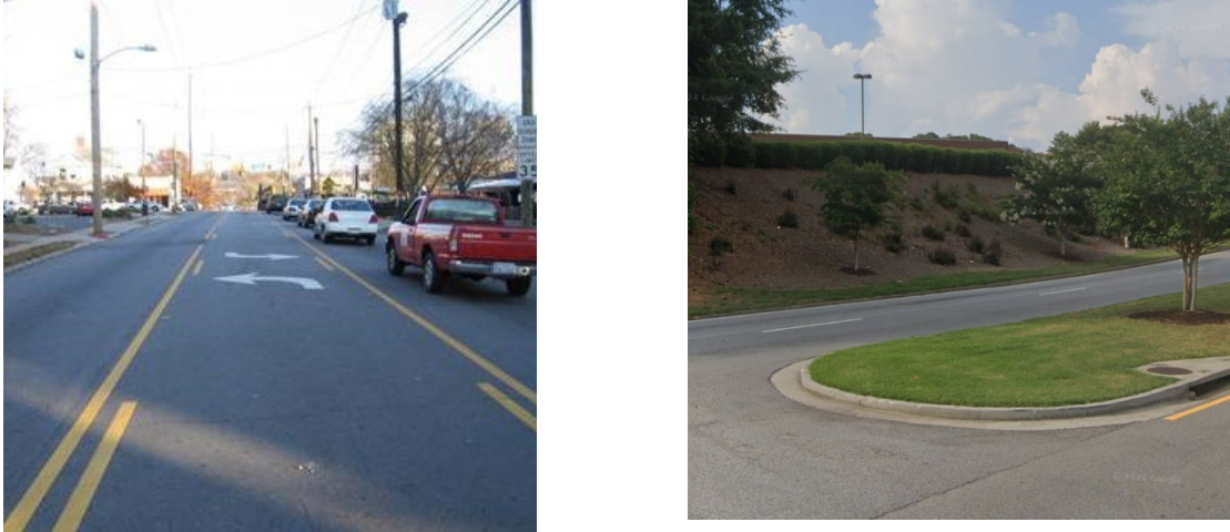
Figure 5: Examples of Center Turn Lanes and Medians
