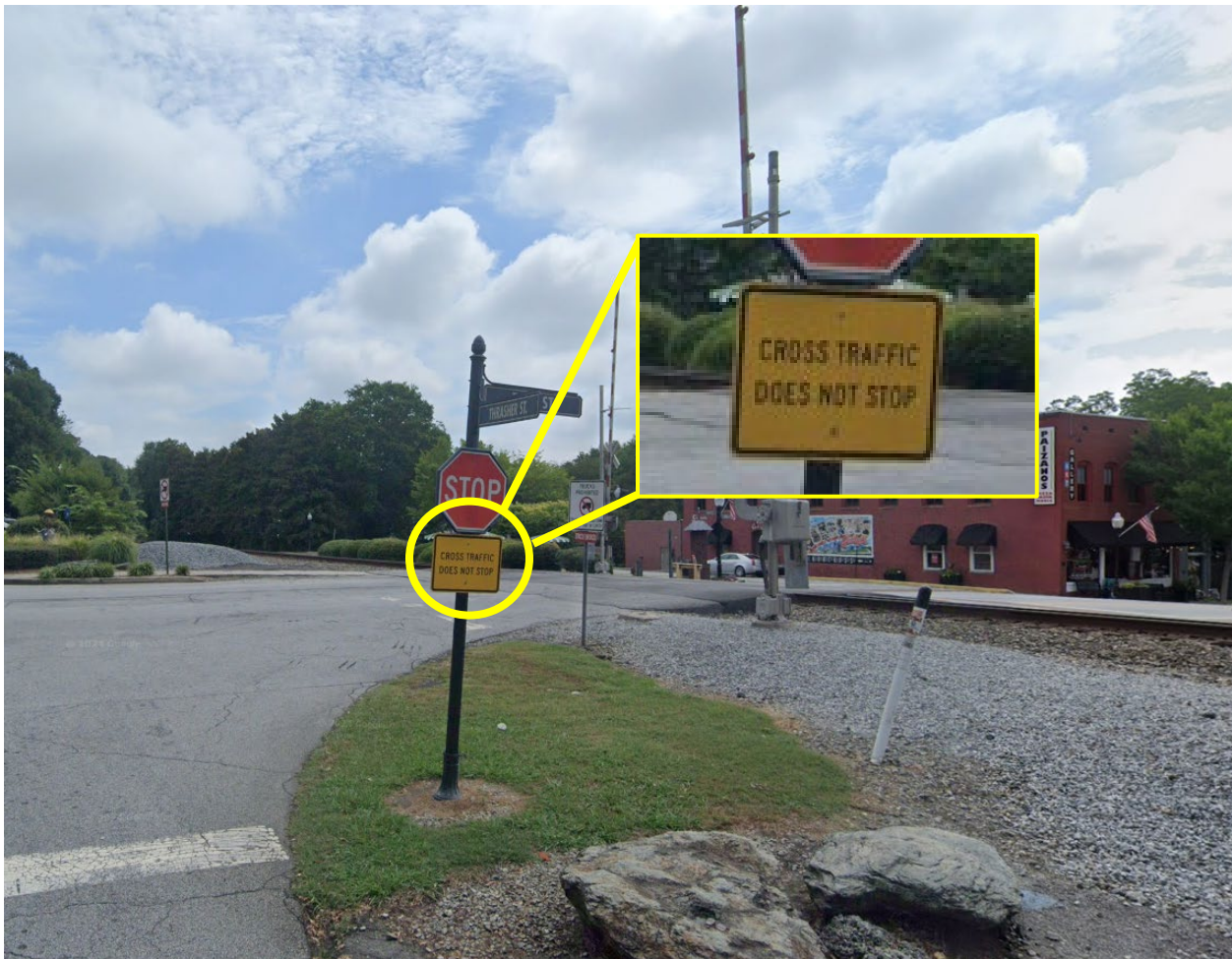
Figure 61: Proper Signage at Stop-Controlled Intersection near At-Grade Crossing
