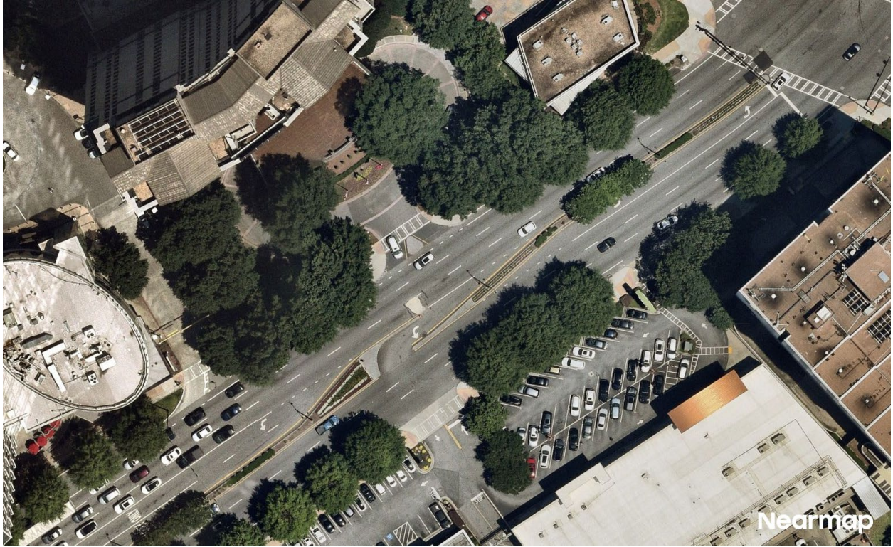
Figure 85: Median Opening on Peachtree Road in Buckhead
