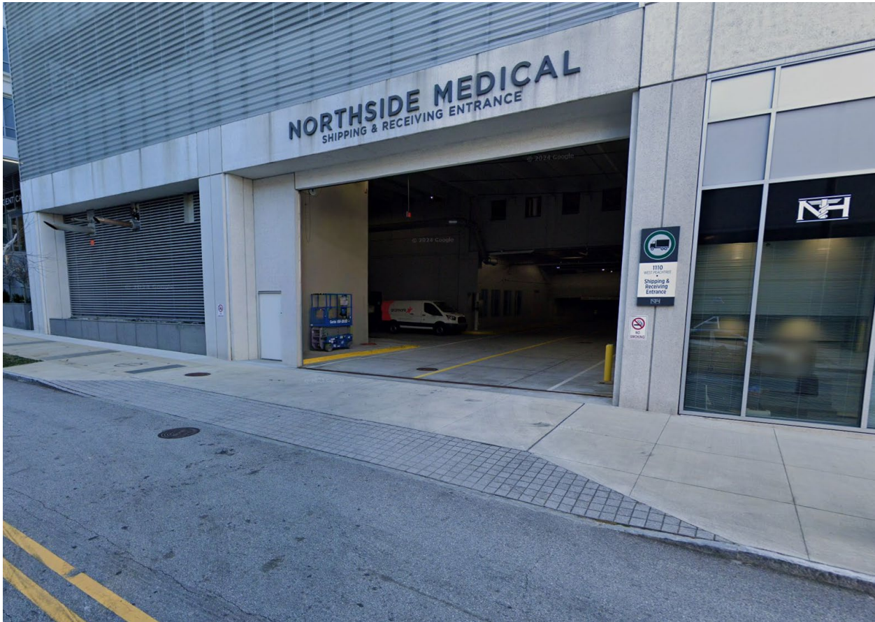
Figure 121: Signed Loading Dock at Northside Medical Midtown
