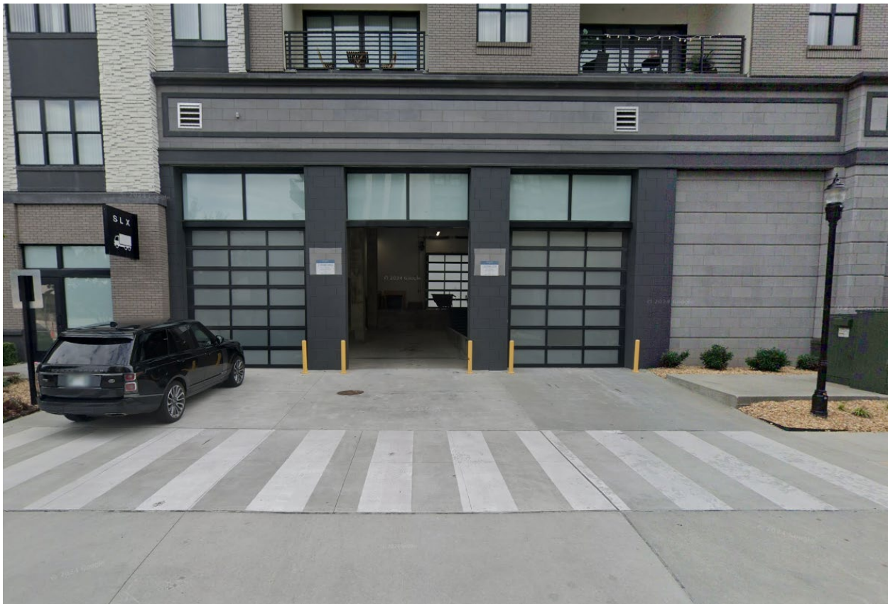
Figure 78: Designed Rolling Door Screen in Chamblee, GA
