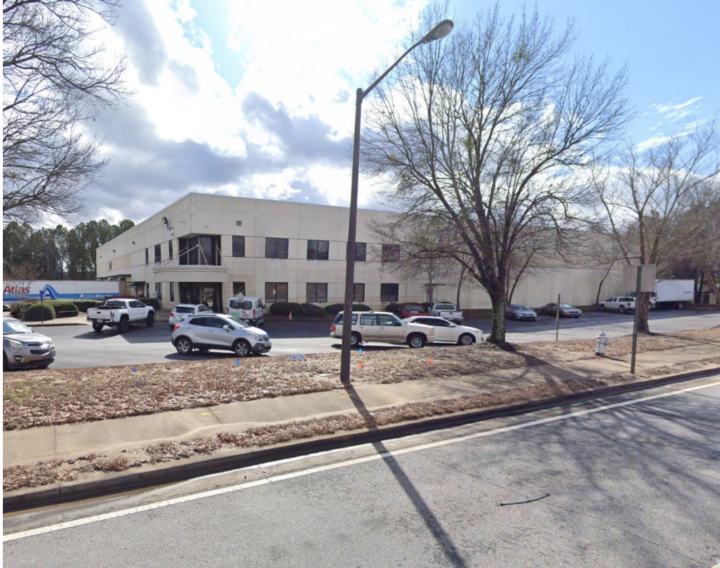
Figure 33: Properly Designed Sidewalk in Mableton, GA
