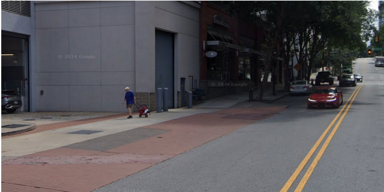
Figure 91: Painted Sidewalk at Loading Dock Entrance, Midtown Atlanta
