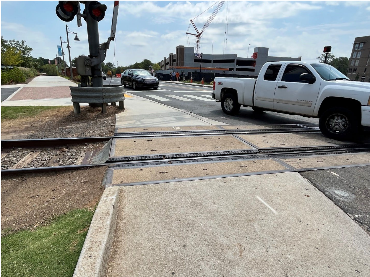
Figure 62: Pedestrian Railroad Crossing on Sidewalk in Woodstock, GA
