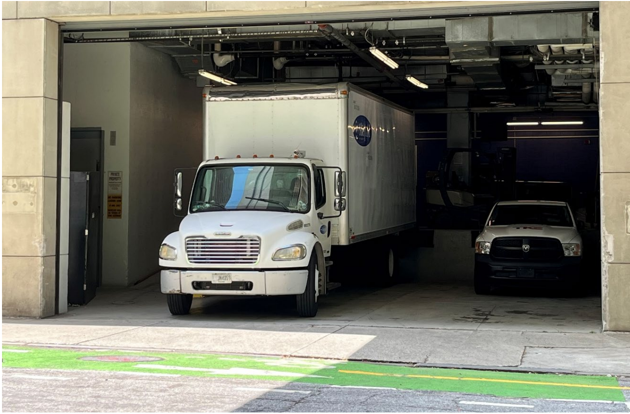
Figure 117: Major Activity Center Buildings with a Flush Dock, Downtown Atlanta
