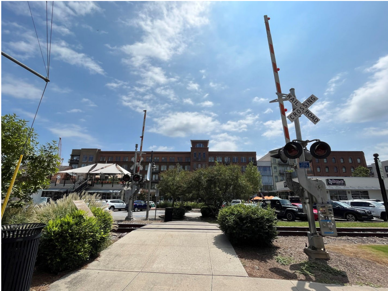
Figure 31: Standalone Pedestrian Railroad Crossing with Pedestrian Oriented Signal and Signage in Woodstock, GA
