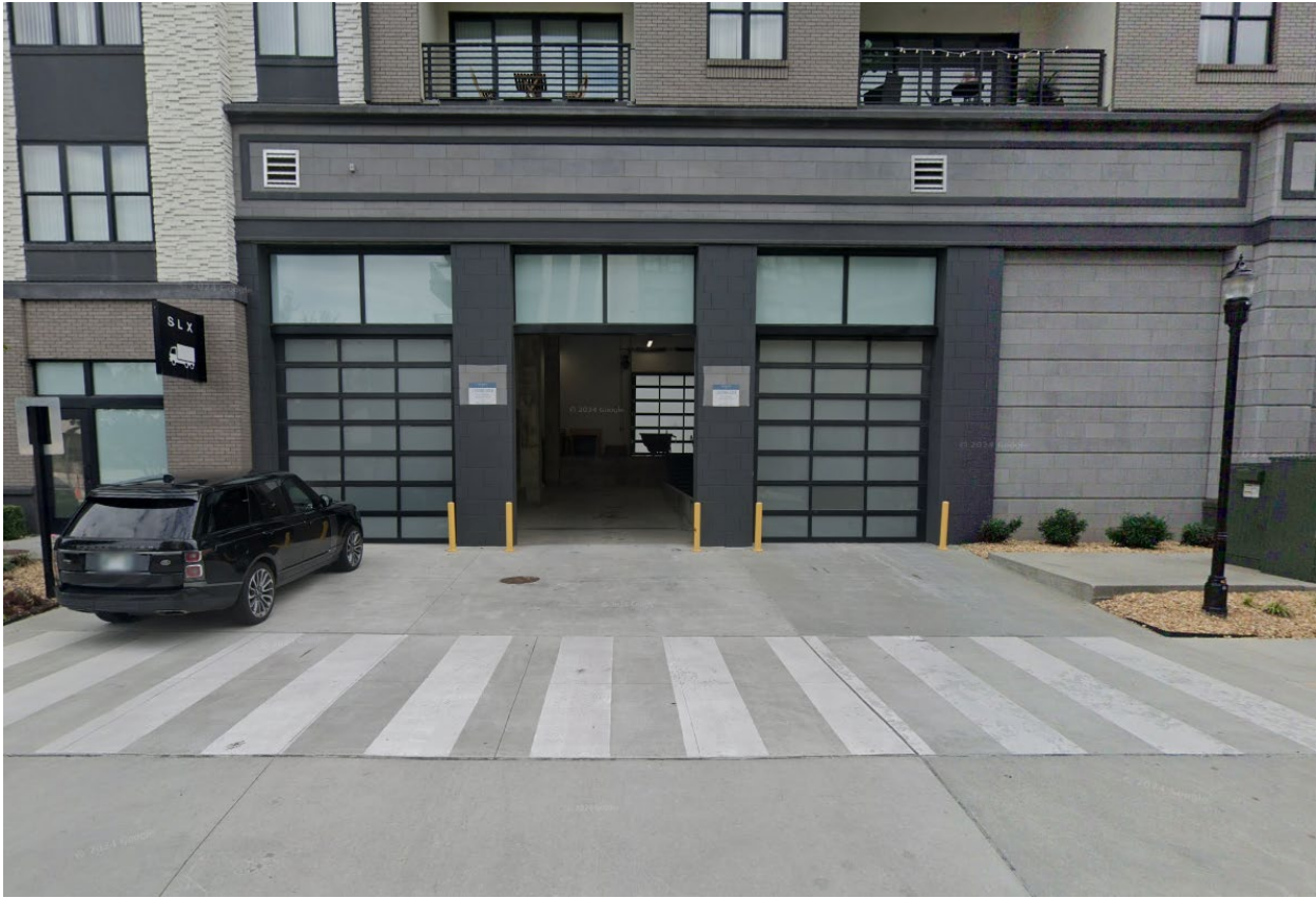
Figure 123: Designed Rolling Door Screen in Chamblee, GA
