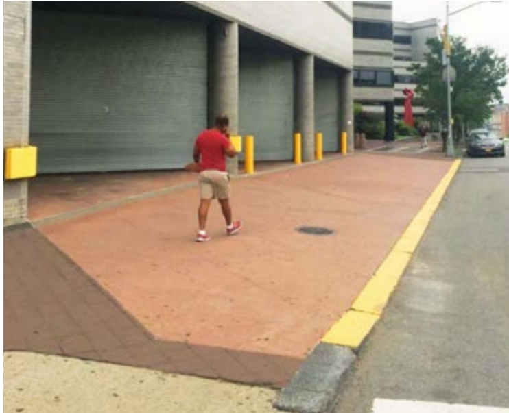
Figure 15: Painted Sidewalk at Loading Dock Entrance
