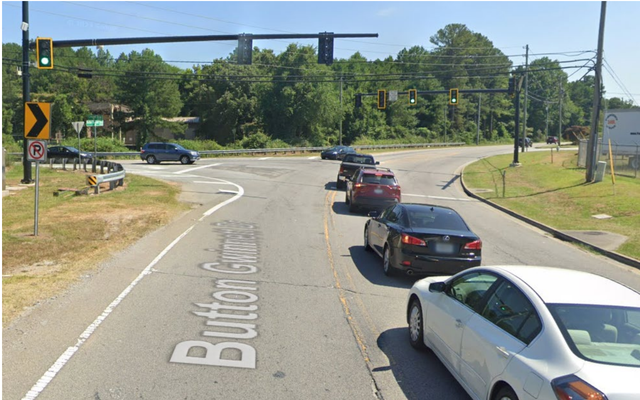
Figure 12: Supplemental Signal Head on Left Supported by Mast Arm
