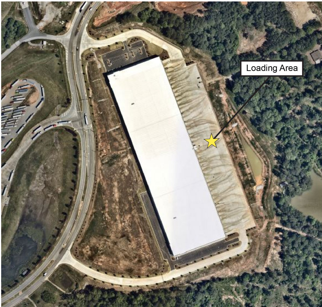
Figure 37: Loading Area Located Away from Roadway
