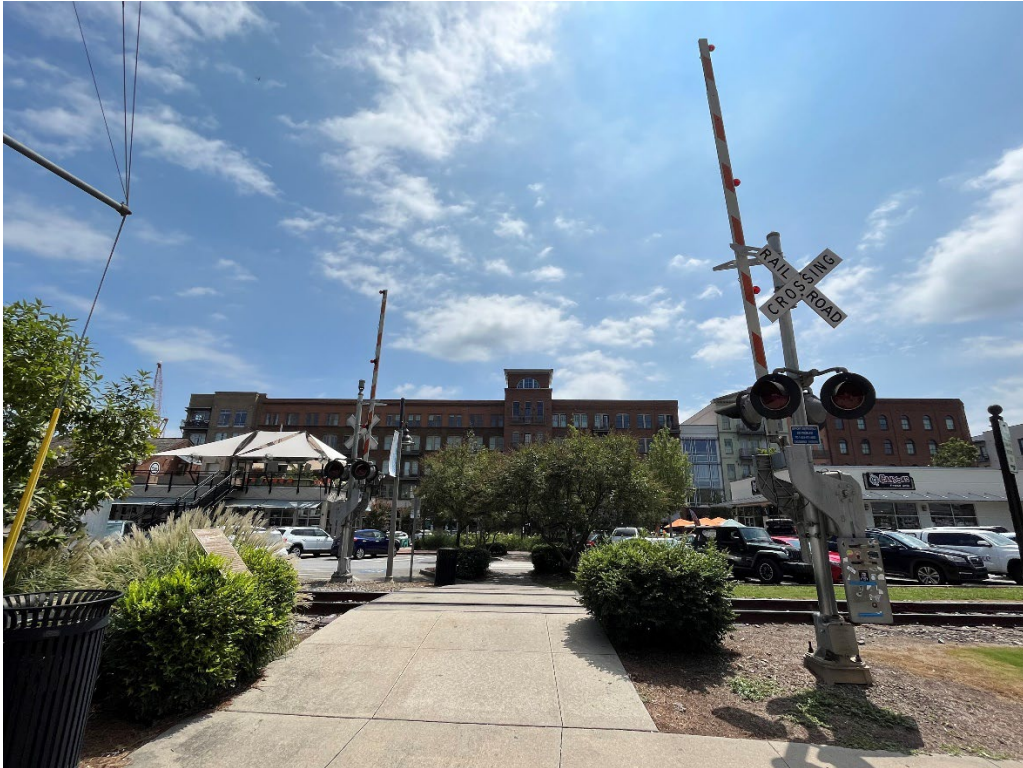
Figure 103: Pedestrian Railroad Crossing with Pedestrian-Oriented Signal and Signage in Woodstock, GA
