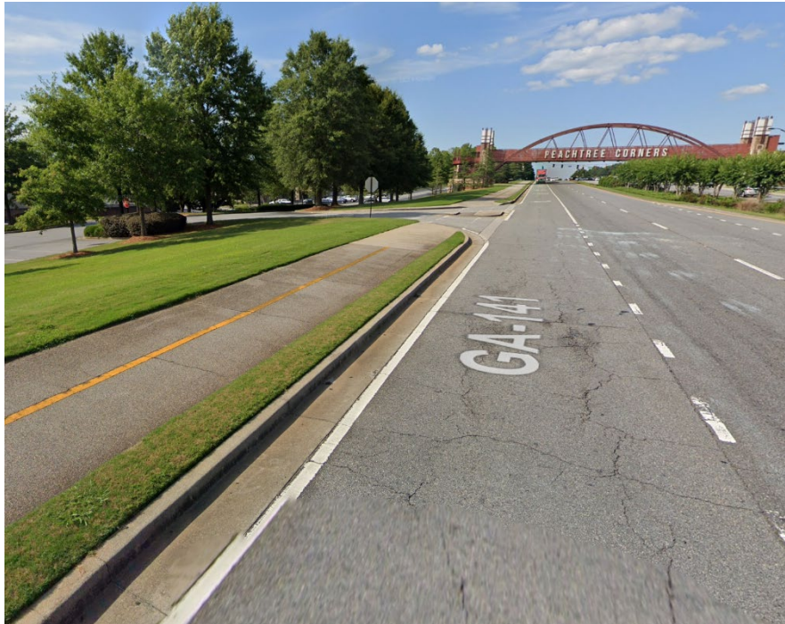
Figure 18: Buffered Multi-Use Path on Peachtree Industrial Boulevard
