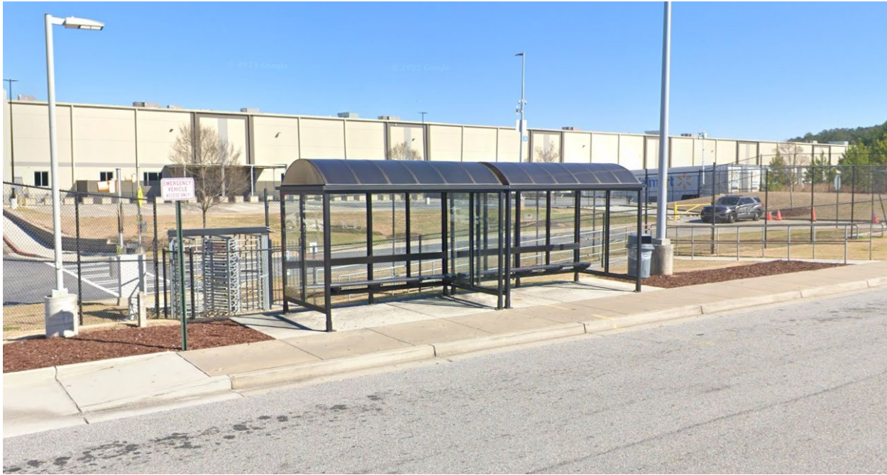
Figure 35: Sheltered Bus Stop with Ramp to Site Entrance
