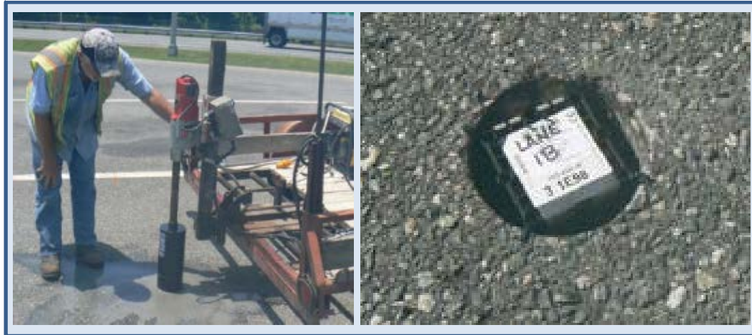
FIGURE 5.4. FDOT TPAS IN-PAVEMENT PUCK DETECTORS
