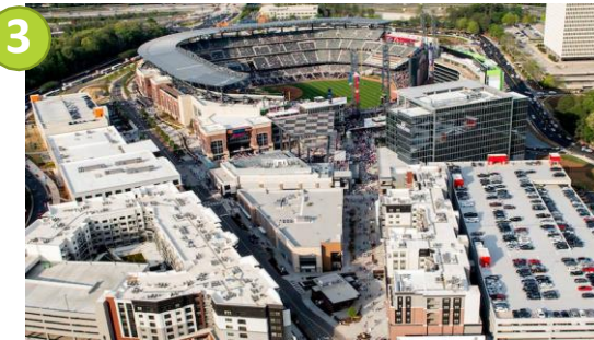
The Battery, Cobb County, GA 1.5M Office SF | 12.7% Vacancy 182K Retail SF | 9.9% Vacancy
