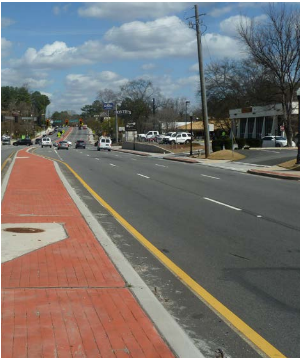
New medians on Buford Highway provide a refuge for pedestrians
