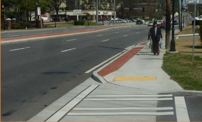
Basic sidewalk infrastructure on major road
