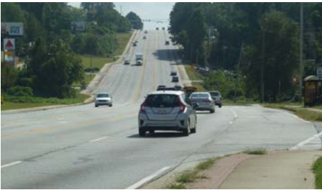
Further north, there are four travel lanes and a center turn lane, speeds remain high, there is inadequate lighting and infrequent (i.e. no) crosswalks despite the presence of transit stops.
