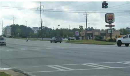
The south end of corridor #1 has multiple risk factors (45 mph speed limit, 6+ travel lanes, inadequate street lighting, moderate demand).
