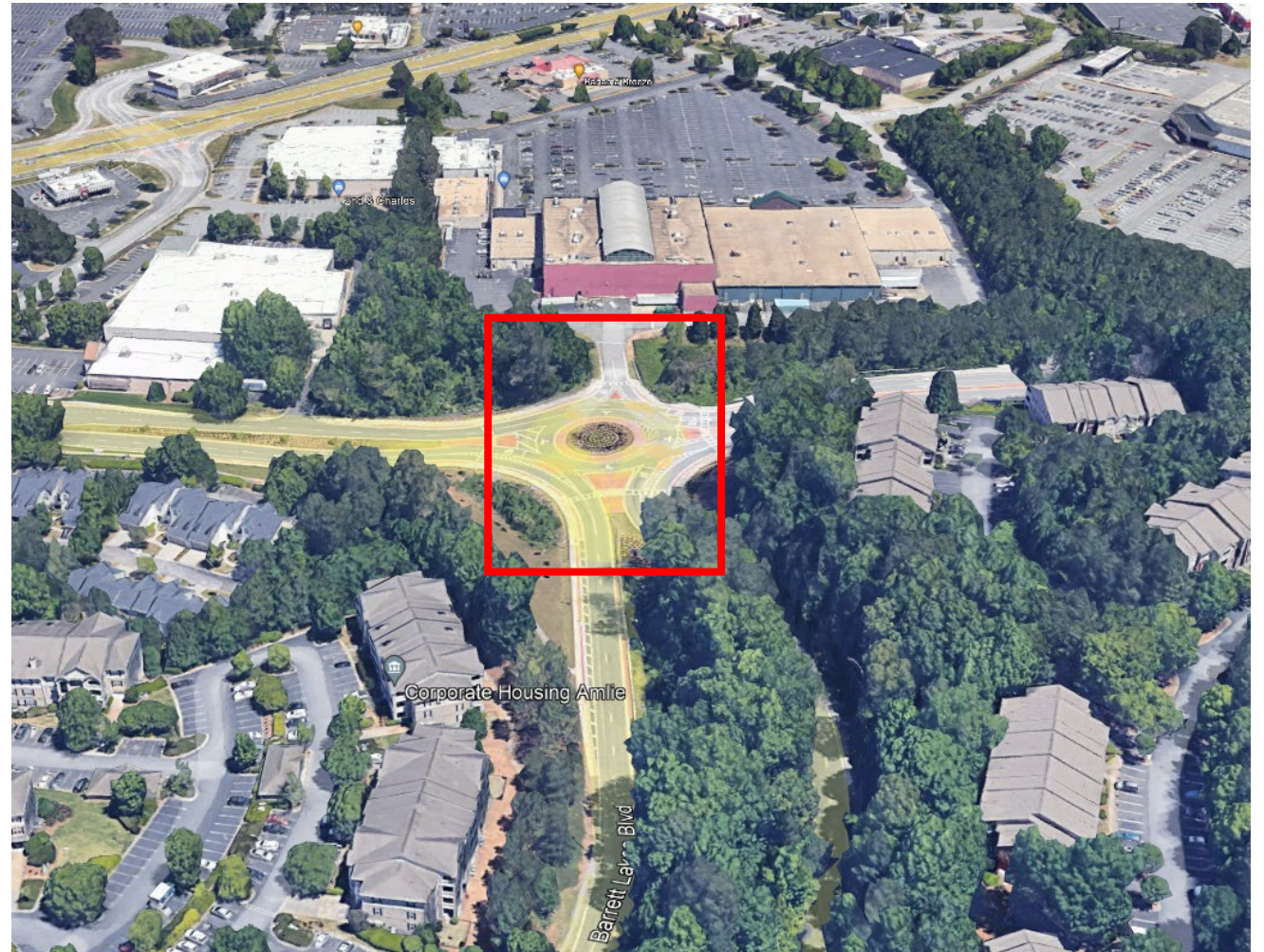
South Barrett Reliever Roundabout (Source: Google Earth)
