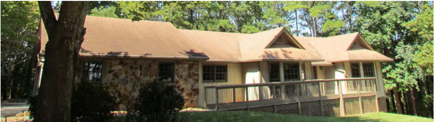
Arts Center East in City of Roswell was submitted to ARC's Green Communities as a Greyfield Site that renovated a residential home into an art gallery and facilities for cooking, painting and clay, wheel, and pottery classes.
