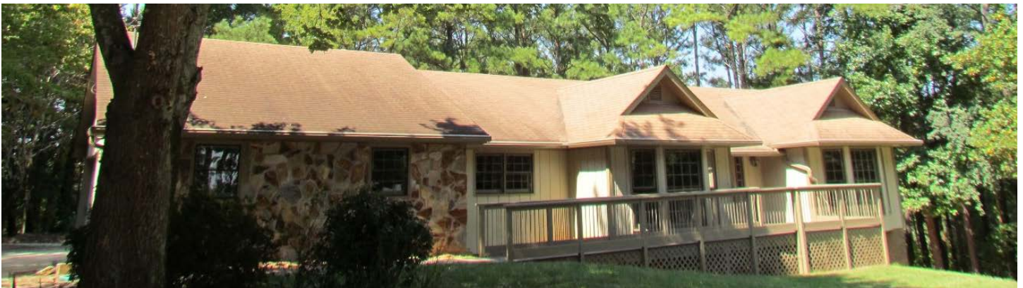
Arts Center East in City of Roswell was submitted to ARC’s Green Communities as a Greyfield Site that renovated a residential home into an art gallery and facilities for cooking, painting and clay, wheel, and pottery classes.
