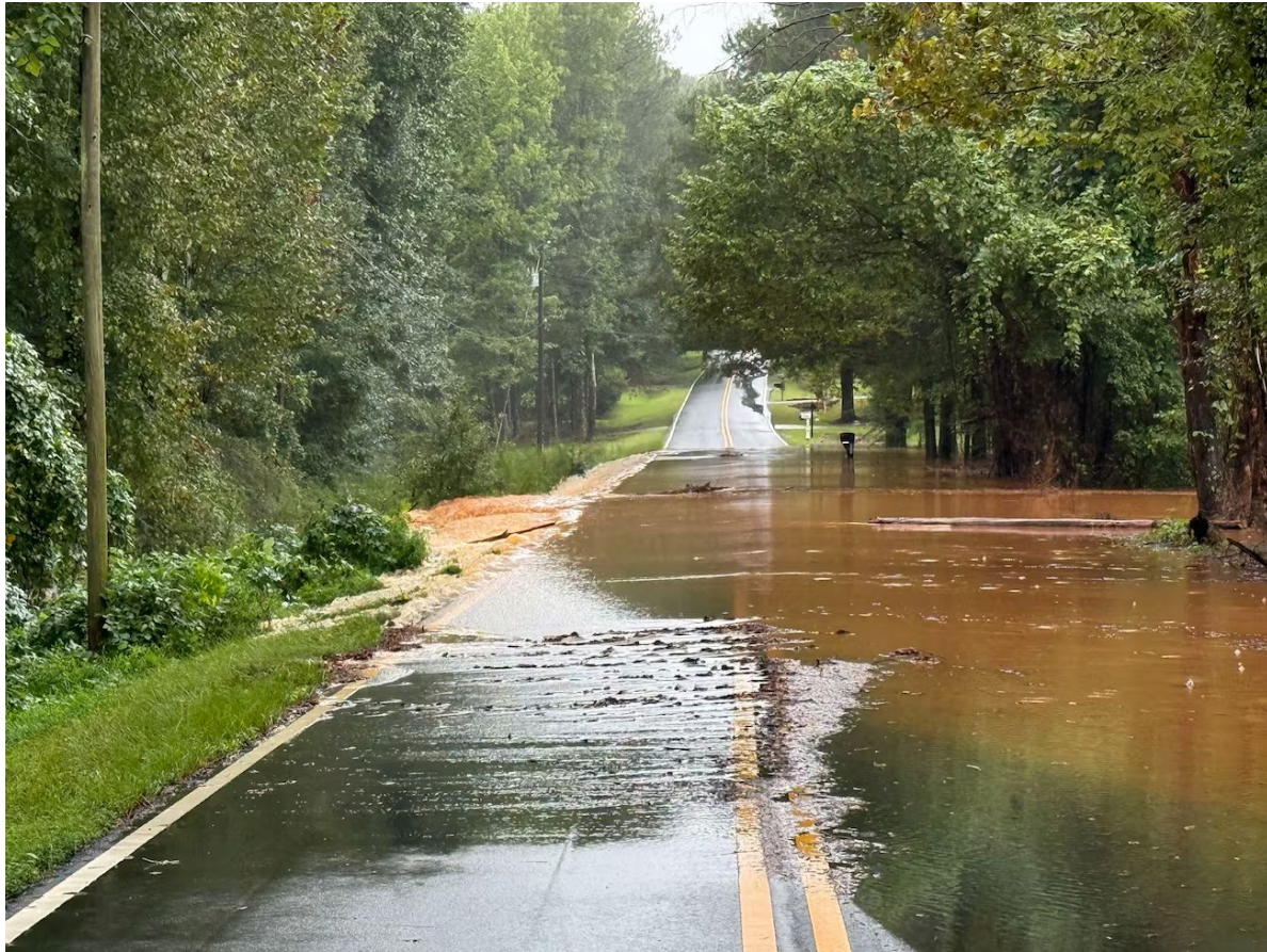
Kinney Lake Road flooding in Carroll County – 12 Sep 2026
