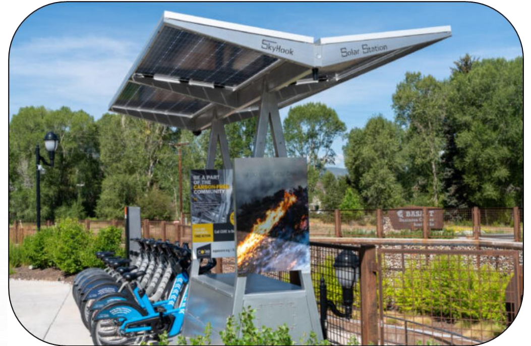
We-Cycle solar-powered off-grid station Aspen, Colorado
