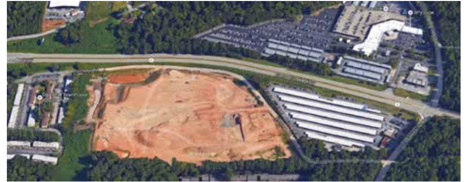
Figure 2.9-1 Aerial of Wally Park redevelopment under construction
