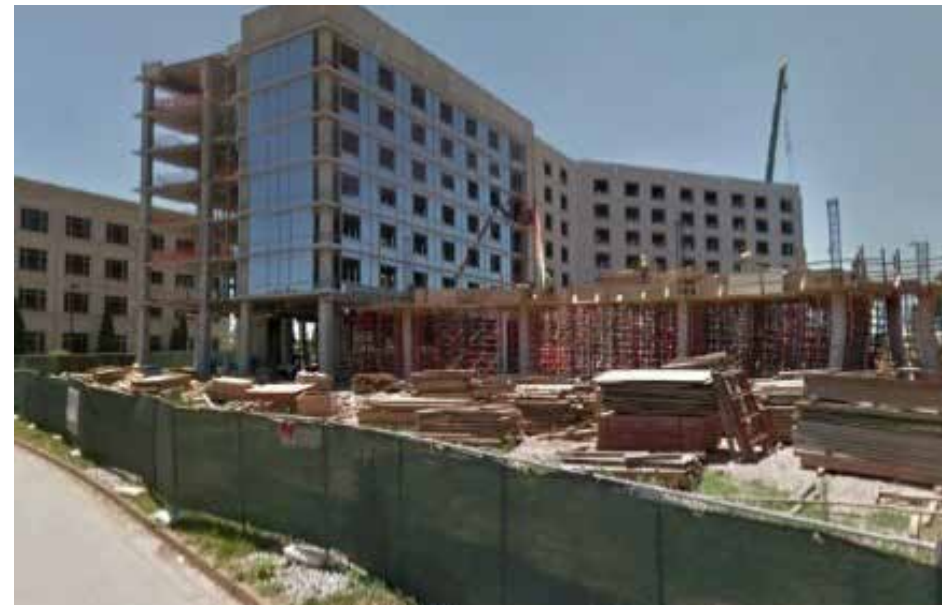
Figure 2.9-11 Gateway Center - Marriott Renaissance Hotel Under Construction
