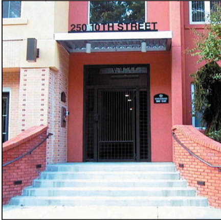
This building provides a secure door into internal hallways, but is not gated from the street.
