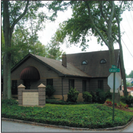
Most buildings in the Study Area are in Standard condition
