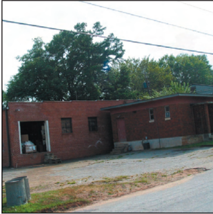
A functional, single-story industrial building typical of the Study Area
