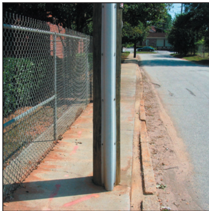
This utility pole's placement creates an unusable sidewalk
