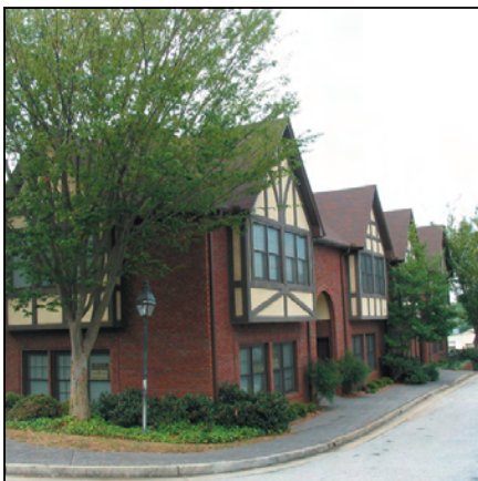
A newer Tudor Revival building on Avondale Road
