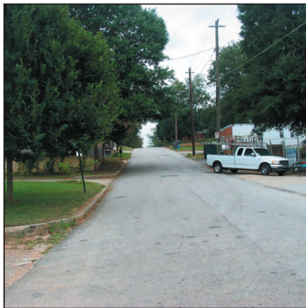
Local Streets, such as Washington Street, are typically 26 feet wide
